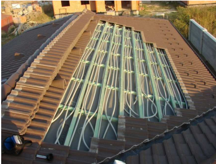
Fig. 8: PP pipes of the ©ISOMAX roof-integrated thermal solar absorber
