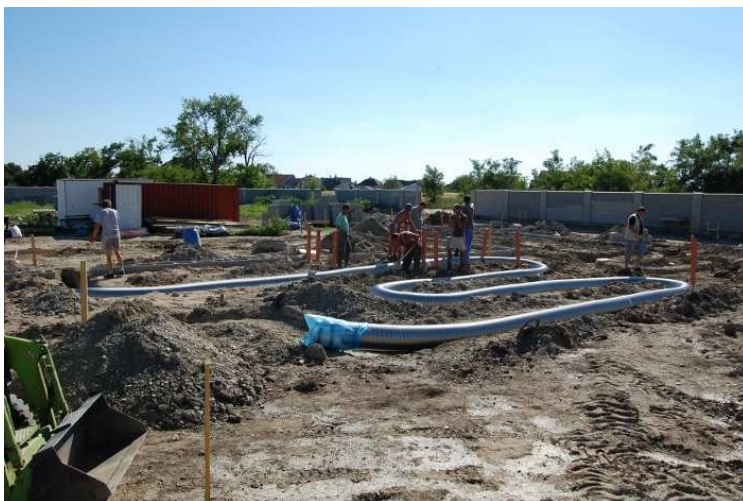
Fig. 9: Laying © ISOMAX Pipe-in-Pipe air heat exchangers
