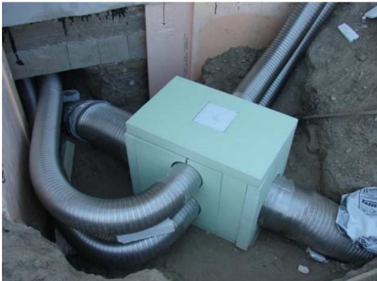
Fig. 10: ®ISOMAX Pipe-in-Pipe summer/winter air heat exchanger.
