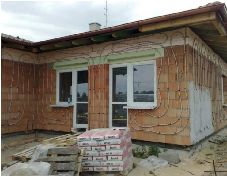
Fig. 7: PP pipes of the ©ISOMAX temperature barrier
