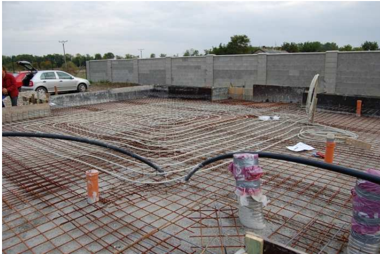
Fig. 6: Construction of the ® ISOMAX heat storage system
