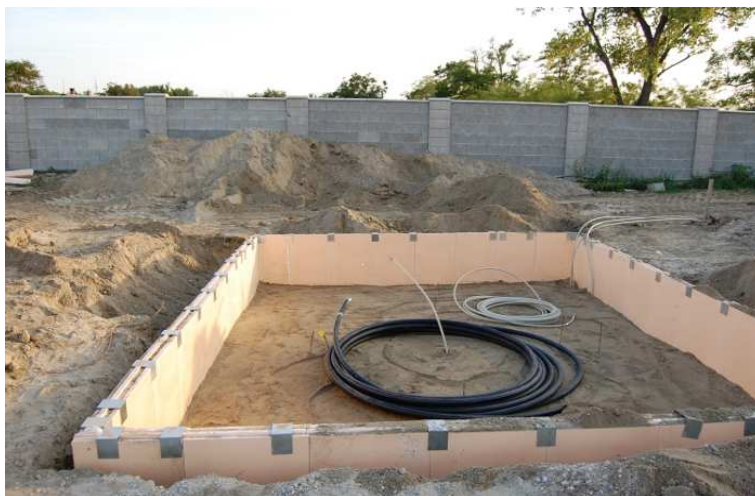
Fig. 4: Construction of an ® ISOMAX core storage system
