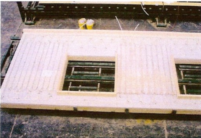
Installation of temperature barrier
