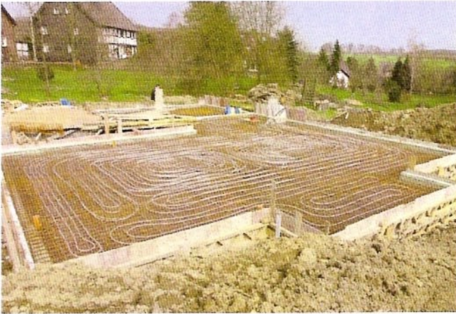
Solid accumulator circuit
